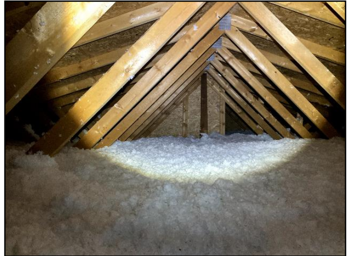
76. General view of attic
