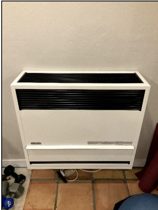
66. Gas space heater
