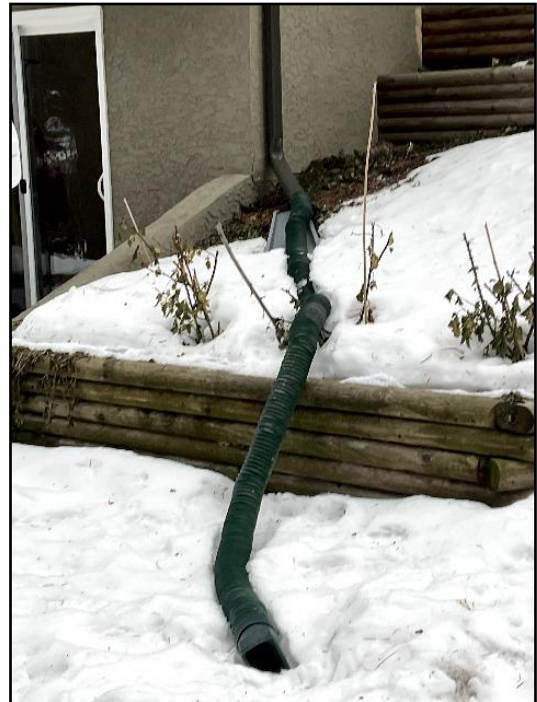
16. Maintain 6 feet from building
