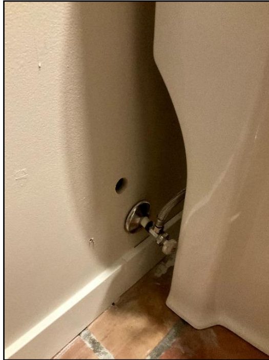
88. Hole drilled near pipe on wall
