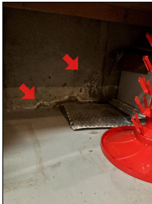
111. Efflorescence
