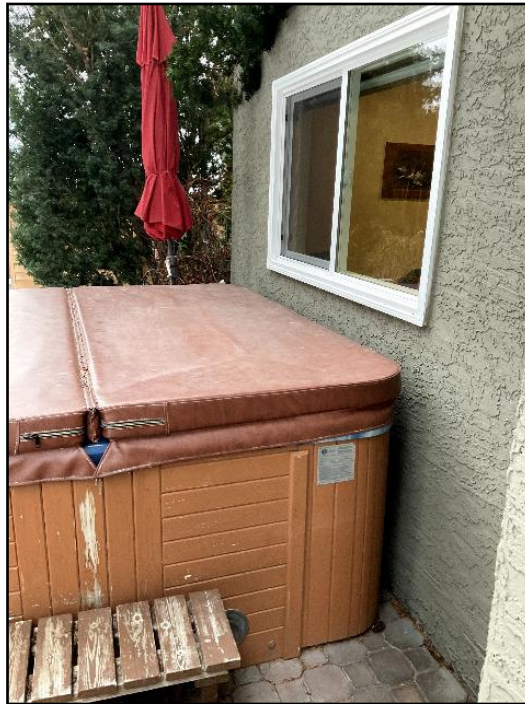
11. Too close to siding
