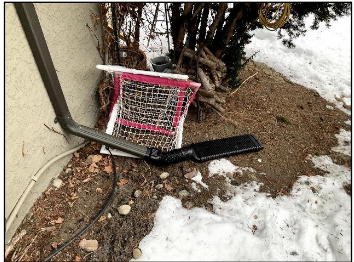
14. Maintain 6 feet from building
