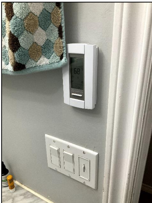
69. Radiant floor heating (electric)
