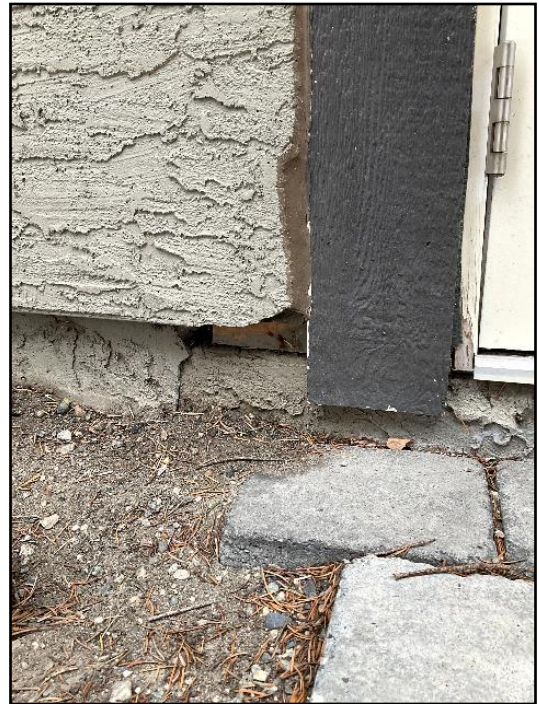
21. Mechanical damage
