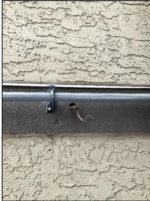
58. Exposed Wires
